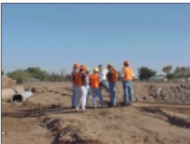
Site visit to Rt. 202 Extension Project in the Phoenix Construction District, Maricopa County. $60 million contract for +/-3.2 miles of highway and structures.
