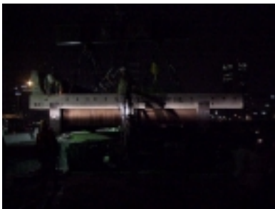
Lane Rental Project at Night Over the James River, Virginia
