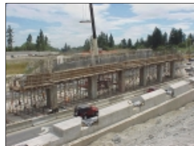
Wisconsin DOT Bridge Construction on the G/I-94 Interchange Project
