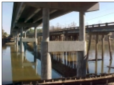
FDOT District 3 site visit to bridge replacement project.
