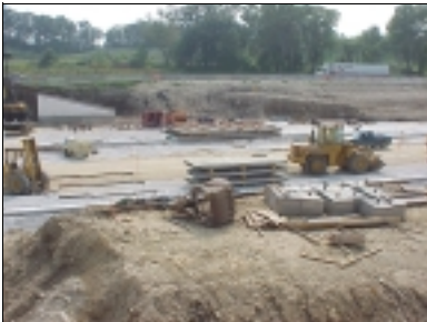
Wisconsin DOT District 2 Site Visit to G/I-94 Interchange Project
