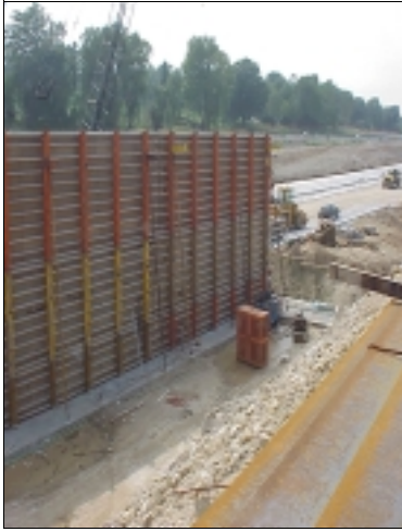
Wisconsin DOT District 2 site visit to G/I-94 Interchange Project.
