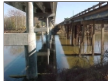
Florida DOT District 3 site visit to bridge replacement project.
