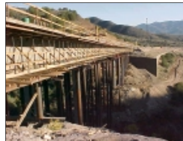
Arizona DOT Rural project site visit. Bridge construction on a new alignment.
