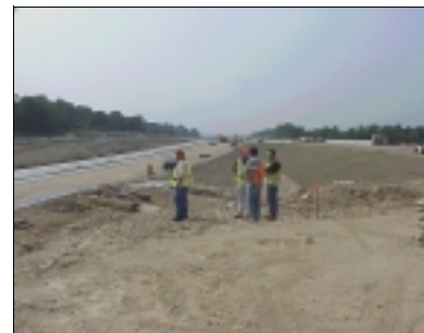
Wisconsin DOT District 2 site visit to G/I-94 Interchange Project
