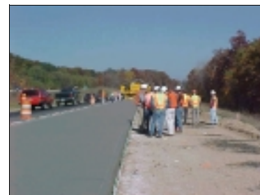
Michigan DOT concrete pavement resurfacing project.
