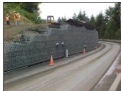
Washington DOT Rural site - emergency project to repair road damaged by landslide.
