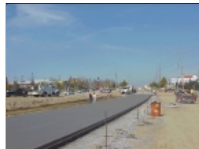
Michigan DOT Concrete Pavement for a New Interchange Project
