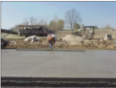
Michigan DOT Rural Project Visit to an Interstate Reconstruction Job
