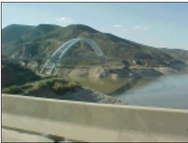
Arizona DOT Bridge at Roosevelt Lake
