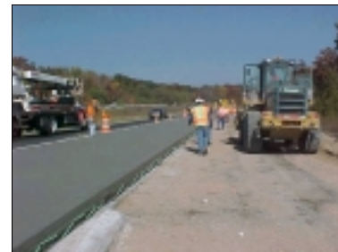
MDOT Concrete Pavement Resurfacing project.
