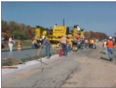
Michigan DOT Concrete pavement resurfacing project
