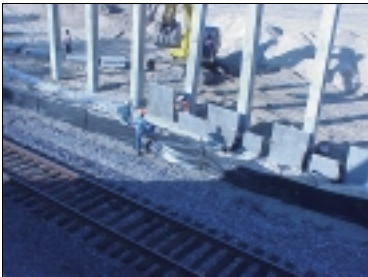
Florida DOT Urban District Construction Project that was Consultant Managed.
