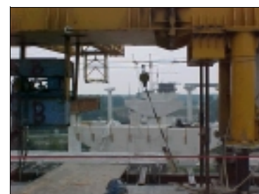
Virginia DOT Launching gantry at Pocahontas Freeway Project
