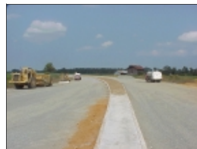
Virginia DOT Fredericksburg District Rt. 3 Project
