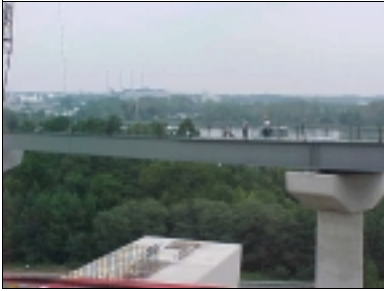
VDOT Pocahontas Freeway Project.
