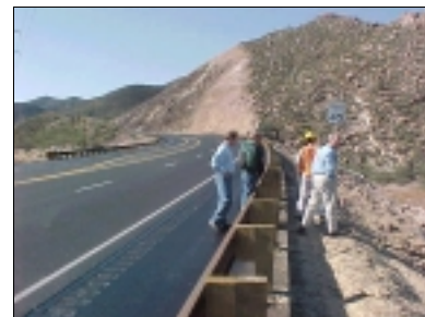
Arizona DOT Newly Widened and Re-surfaced Rural Road
