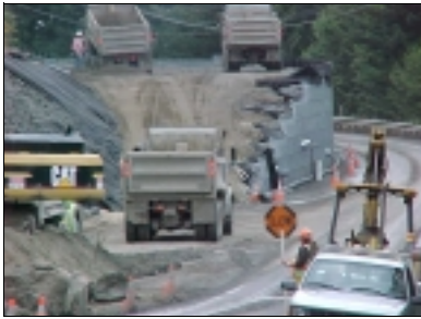
Washington DOT rural site - an emergency project to repair road damaged by landslide
